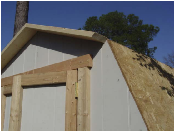
Installing the Fly Rafters
