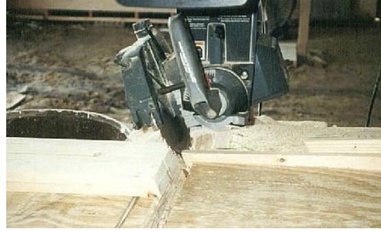
Sawing the fly rafters
