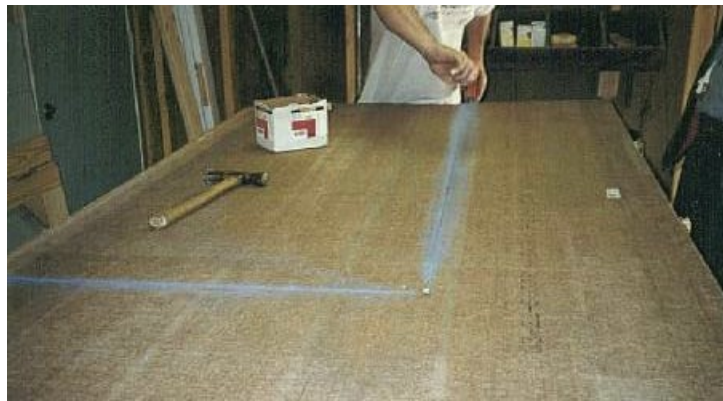
Cut through the back of the siding at the top and side of the door.
