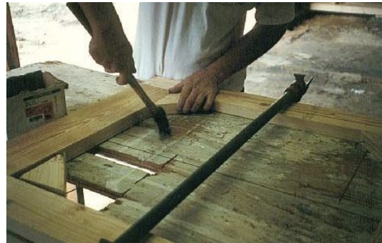
Nail the corner blocks in place.
