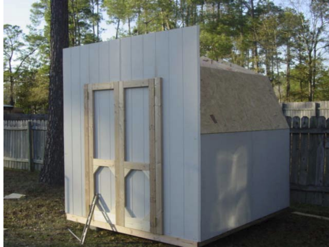
Attach siding with door assemblies on the front.
