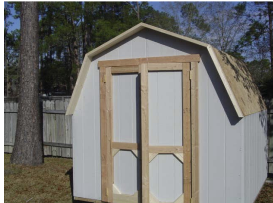
Front Fly Rafters Installed
